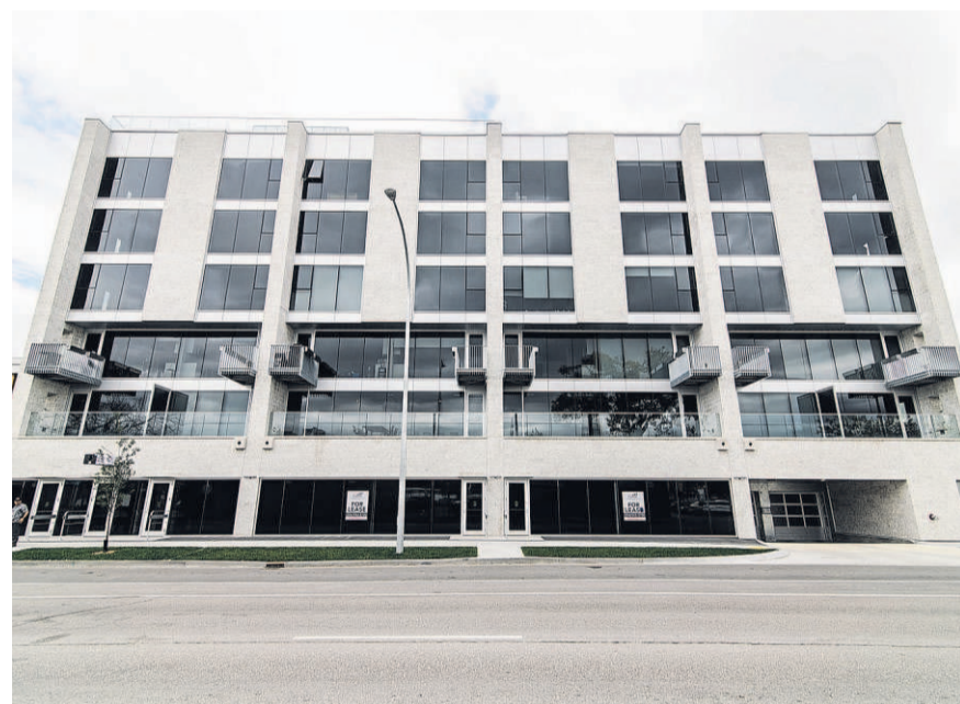
The exterior of Sherbrook Flats is clad in local Tyndall stone limestone from Gillis Quarries.
